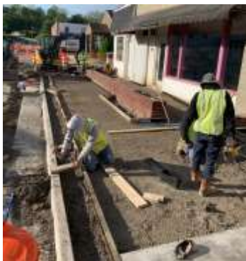
Phase 3A/B Construction Before.....
